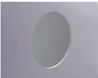
One hole to cut.
